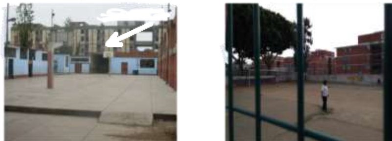
Figure 19. Example of poorly maintained basketball courts
