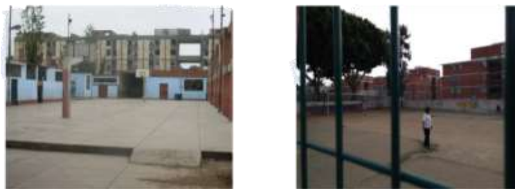
Figure 26. Example of poorly maintained basketball courts
