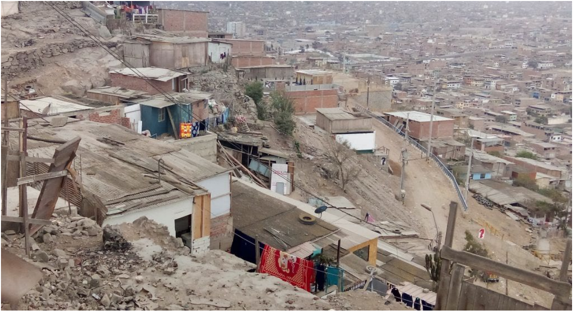
Figure 4: Lack of adequate infrastructure in Villa El Salvador https://intrepidtimes.com/2022/12/a-world-apart-in-villa-salvador/
