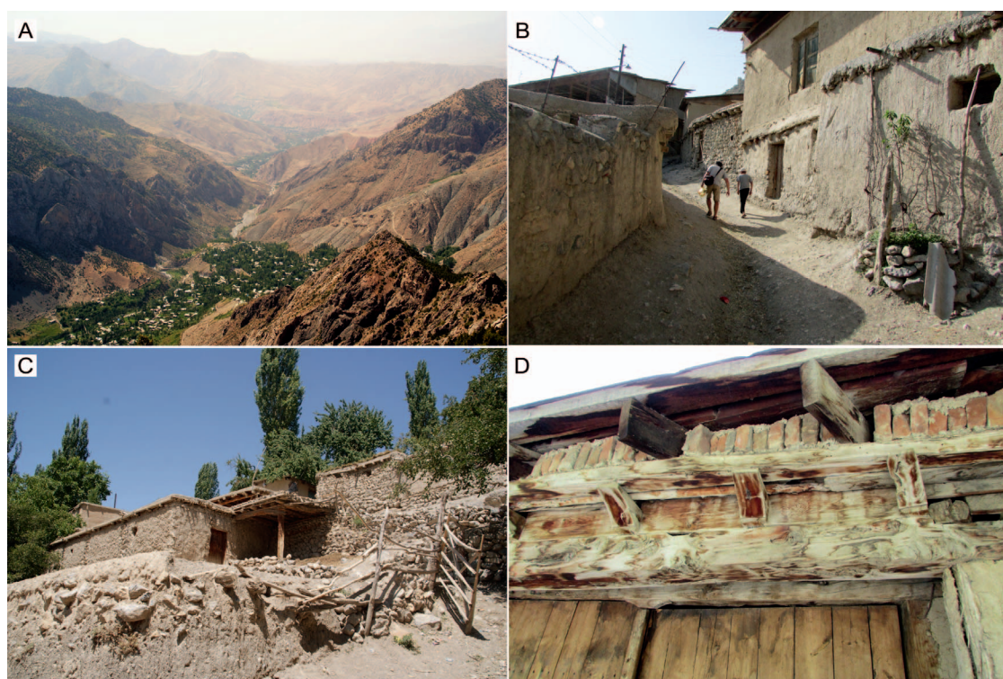
Figure 2. (A) General view of the Artuch village, situated within alluvial cone of small right tributary of the Urech River. (B) and (C) Typical traditional buildings of the central part of the village. (D) Construction elements made of juniper wood.
