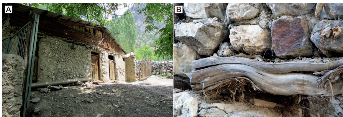
Figure 5. “Cottage #2” site. (A) The stony outbuilding with an “attic” for storing hay. (B) Wooden construction elements within stone wall.
