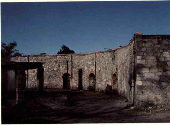
Figure 5. The ovens (los hornos) used for processing the Maguey Verde occupy this stone structure. The cabezas are fed in through the arched entryways.
