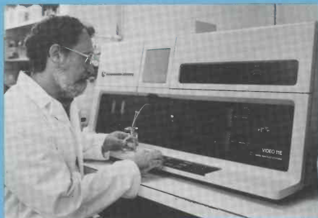
John McGrady uses a spectrophotometer to evaluate nitrate levels in lettuce.
